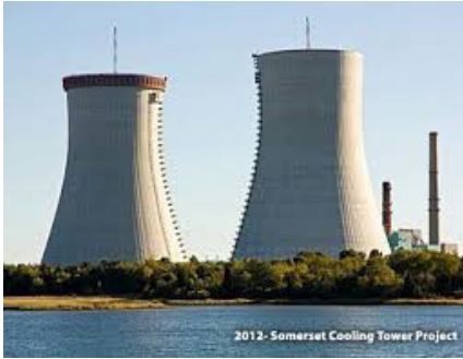
Concrete power station cooling towers
