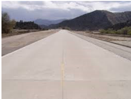
A concrete road
