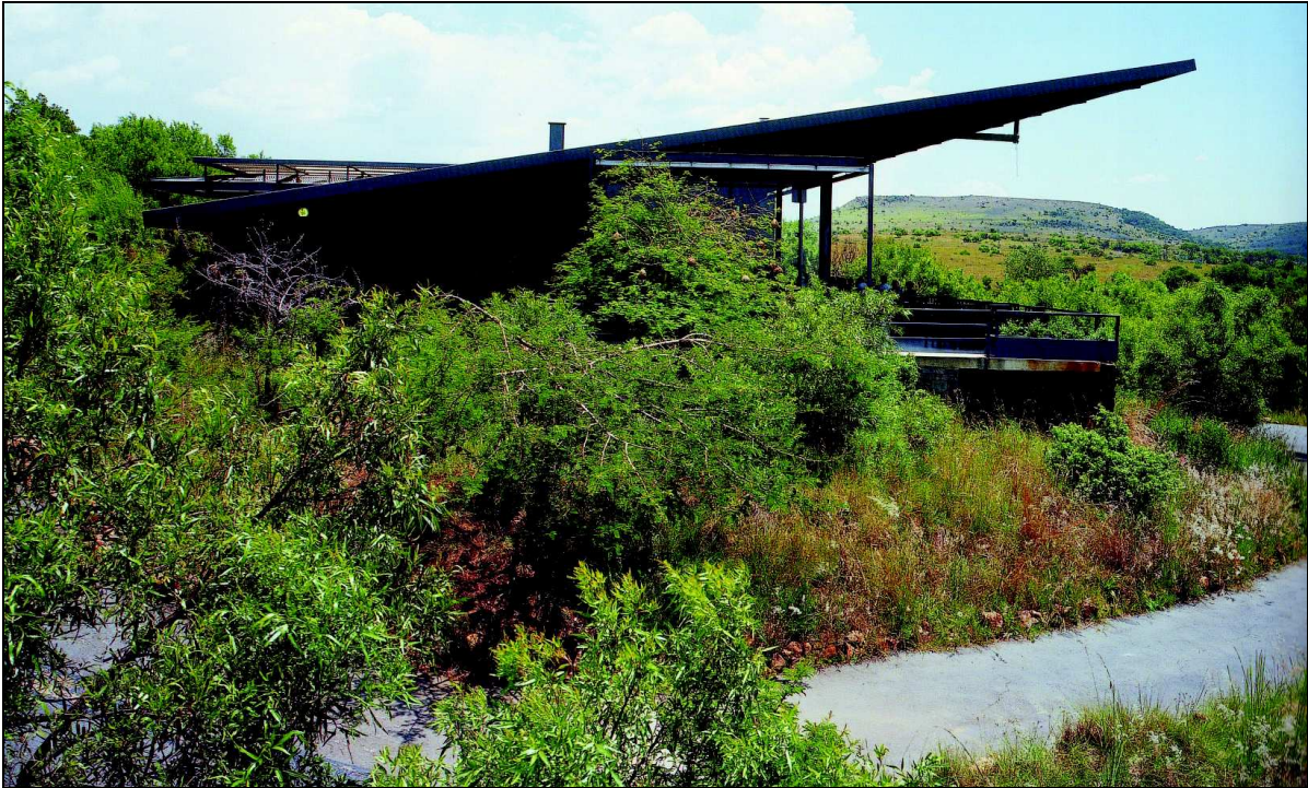
Figure 10a: Cradle of Humankind, Restaurant , Gauteng. Daffonchio Architects & Associates.
